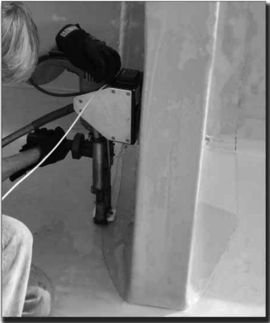
An operator uses a thermoplastic hot gas/hot air extrusion welding machine to join PVC lining sheets. Photo courtesy of Curtis Goad.
